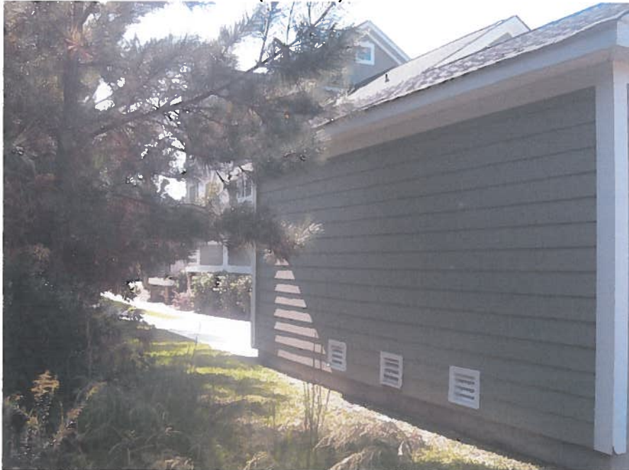
GARAGE RIGHT SIDE VIEW (10-30-07)
