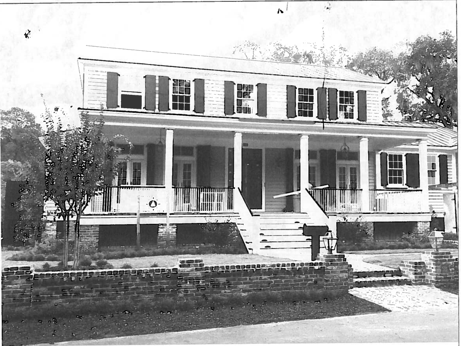
FRONT VIEW (SEPT 26 2013) 505 EAST STREET
