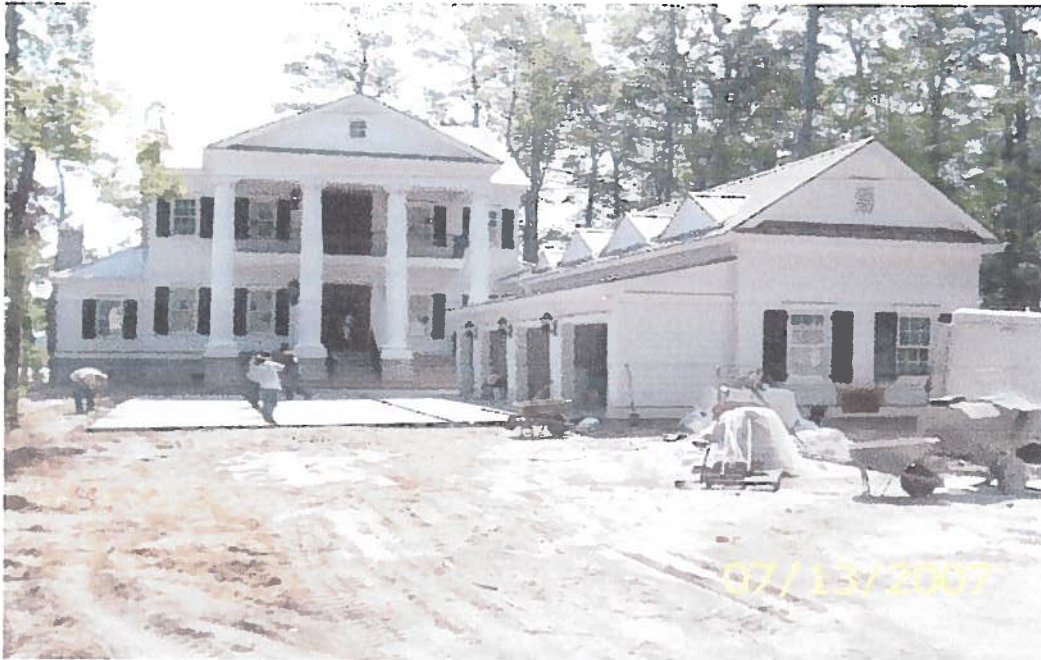
33868 FRONT GARAGE VIEW
