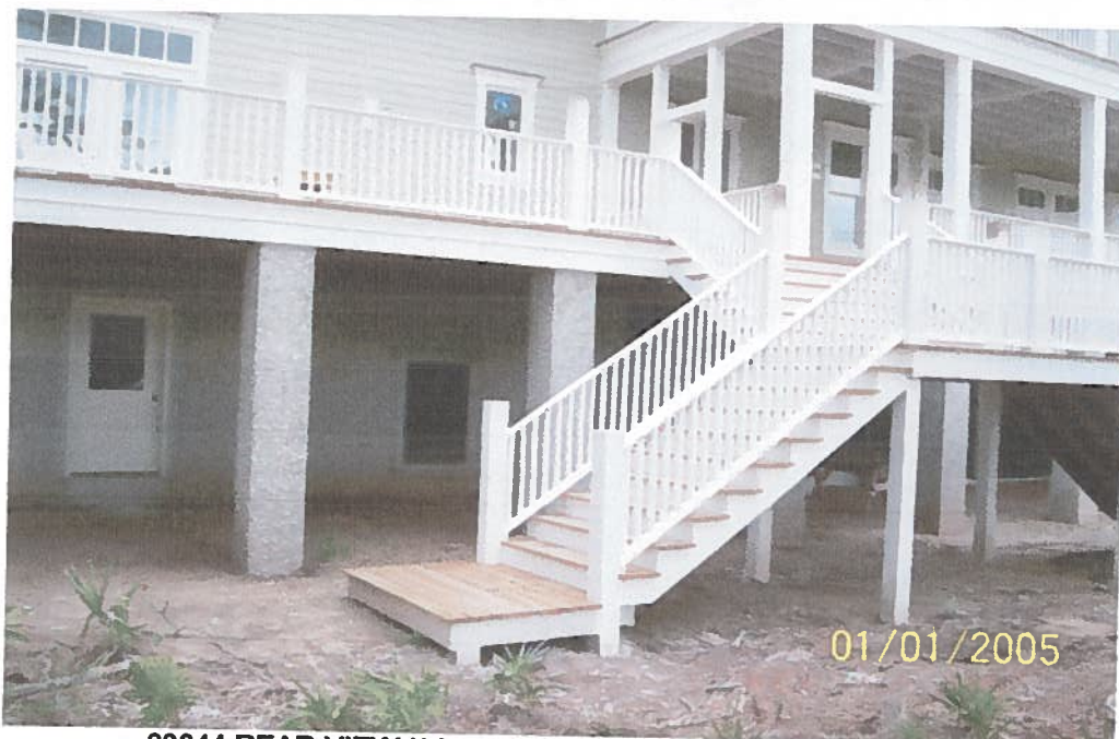
33844 REAR VIEW **date on picture incorrect, should be 7/3/07
