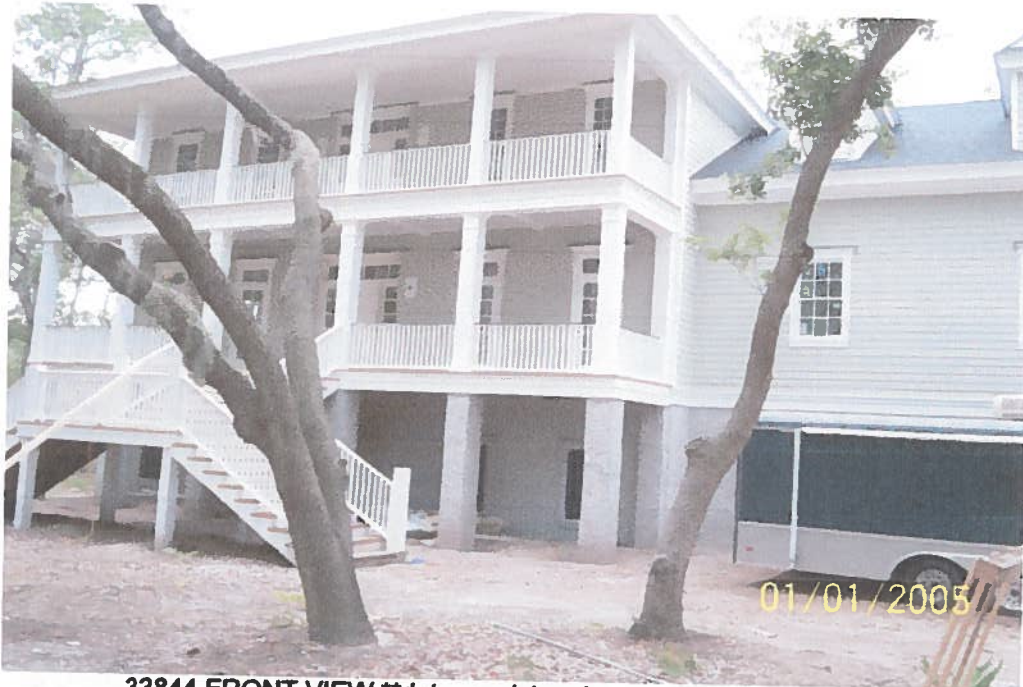
33844 FRONT VIEW **date on picture incorrect, should be 7/3/07
