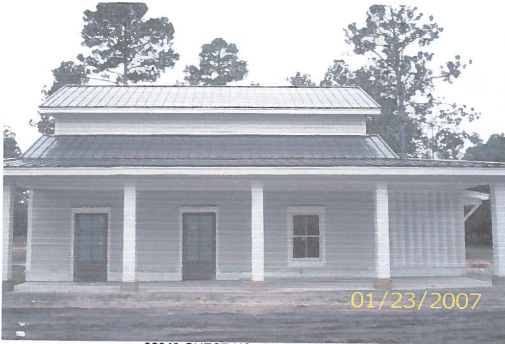
32940 GUEST HOUSE FRONT VIEW
