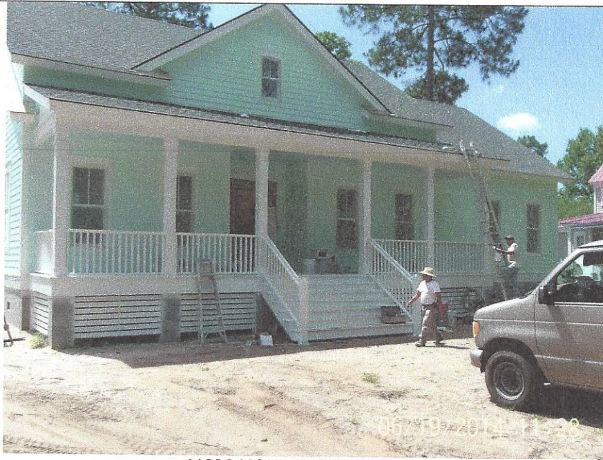
41886 HOUSE FRONT VIEW
